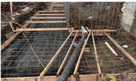
Rebar at Retaining Wall Roofing
