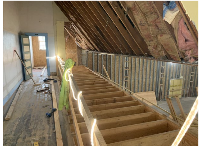
Level 2 Mezzanine Floor Infill
