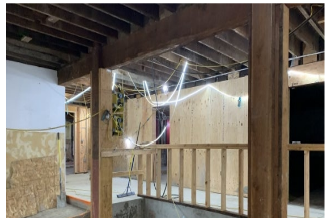
Basement Pony Wall Framing and Concrete
